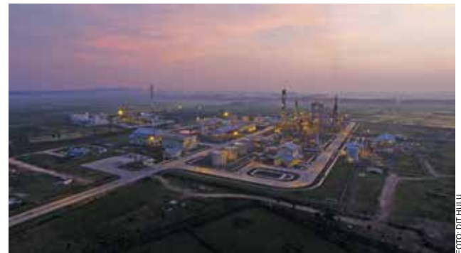
Central Processing Plant (CPP) Gundih, PEP Asset 4 Cepu Field.
