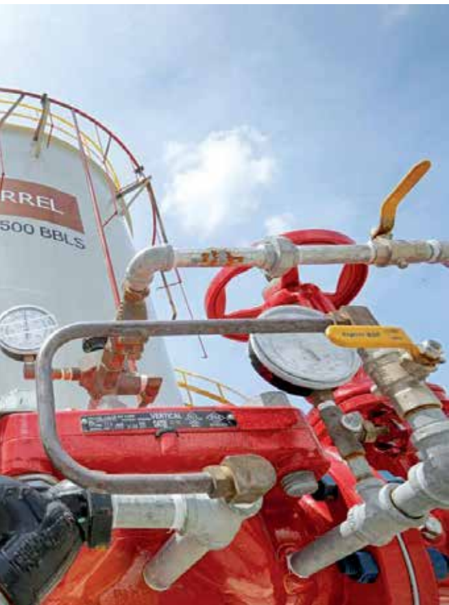
CO2 Removal in one of the Java Subholding Upstream Regional operating fields.
