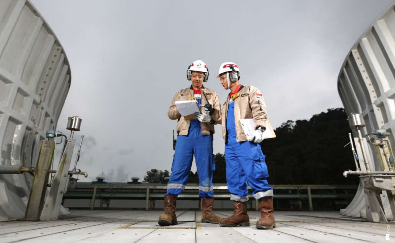
Sejumlah Pekerja sedang melakukan pengecekan di Cooling Tower area Karaha. A number of workers are checking at the Cooling Tower in the Karaha area.
