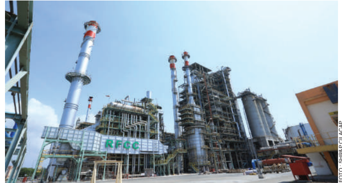
Unit Residual Fluid Catalytic Cracking (RFCC) Plant Cilacap.
