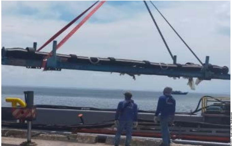
Proses pergantian pipa bawah laut/ subsea hose .
