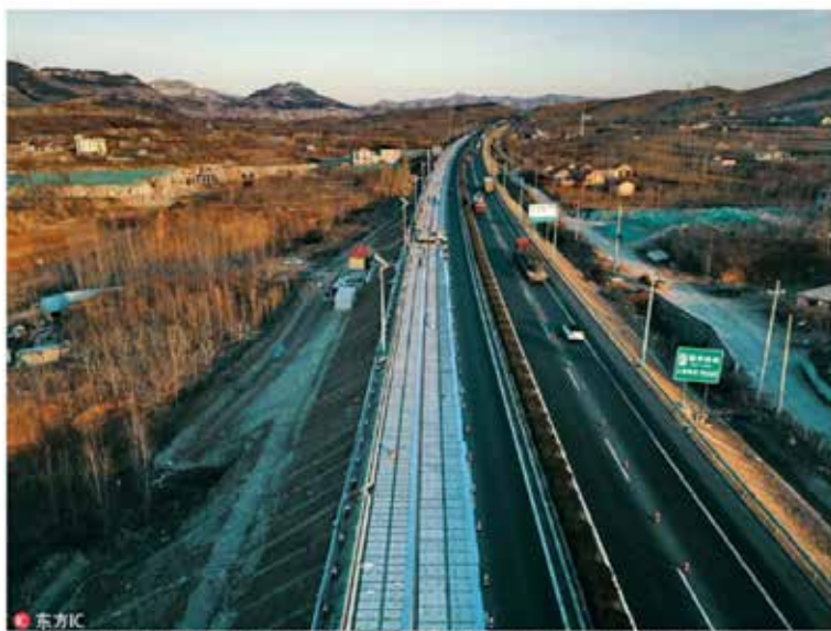
China's photovoltaic highway set to generate 1 million kWh of electricity per year. Image: People's Daily Online
